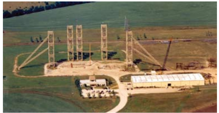
EPRI's former transmission tower test facility in Dallas, Texas.
