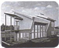
Not only does the roof's extension beyond the southern wall increase shading, it gives the home a definite style. Photo by Gayle Babcock, Architectural Imageworks.
