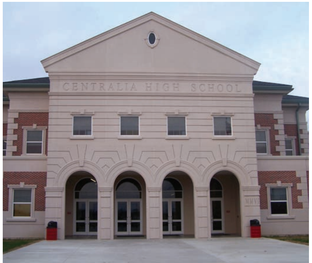
Centralia High School, Centralia, Ill. PHOTO COURTESY OF GATE PRECAST
